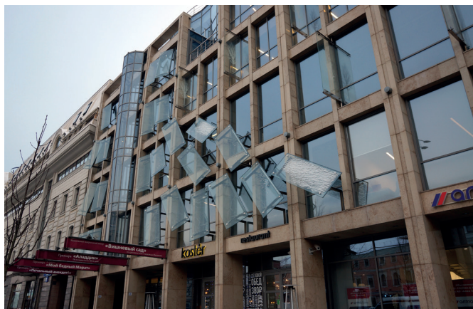
Fig. 2. The façade of the mixed-use complex featuring flying window glasses. The building accommodates the Cherry Orchard Moscow Theatre Centre
